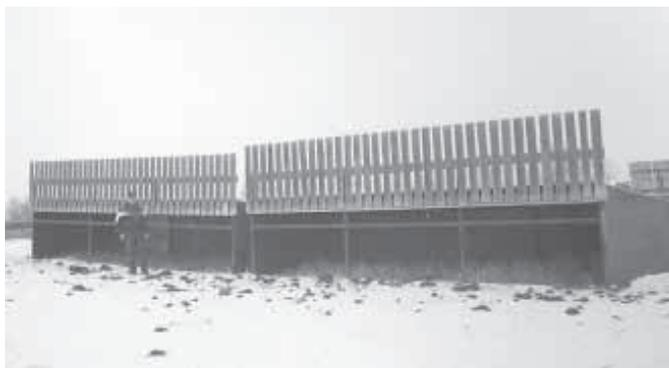
Windbreak extends about 3 ft. above shelter's roof to keep wind from blowing down right in front of shelter.
