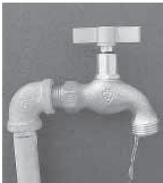
"No freeze" faucet starts to drip automatically when temperature drops below 34 degrees Fahrenheit.
