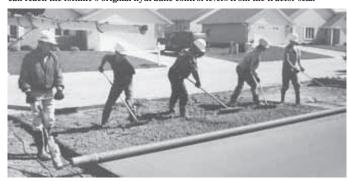
Spin Screed uses a heavy duty right angle drill to rotate an aluminum pipe (above). Pipe is laid over the poured concrete and then pulled along the surface opposite the direction pipe spins. Spinning pipe levels high spots and fills low spots in front of it. Drill is mounted in a specially designed "T" handle to make it easy to use (right).
