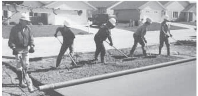
Spin Screed uses a heavy duty right angle drill to rotate an aluminum pipe (above). Pipe is laid over the poured concrete and then pulled along the surface opposite the direction pipe spins. Spinning pipe levels high spots and fills low spots in front of it. Drill is mounted in a specially designed “T” handle to make it easy to use (right).
