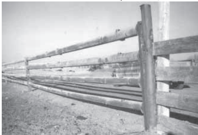
"Moveable" corral consists of big 6 by 38-ft. panels that are made from center pivot irrigation pipe and channel iron.
