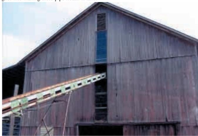
Barnosky removed vertical wood siding to make an opening about 32 in. wide from top to bottom of his barn. He then installed a line of removable windows in opening.
