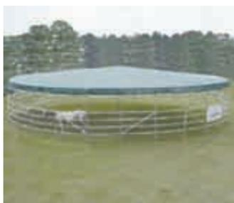
Build-it-yourself, 50-ft. dia. covered riding ring bolts together quickly and costs less than \$3,000.
