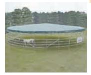
Build-it-yourself, 50-ft. dia. covered riding ring bolts together quickly and costs less than \$3,000
