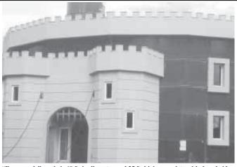
"Farm-made" castle is 60 ft. in diameter and 25 ft. high, complete with drawbridge. Four heaters mounted on central support heat the large structure.
