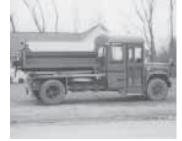
To shorten the bus, Fry slid the wheels up and cut off part of the driveshaft. Then he cut 17 ft. off the frame on the back end.
