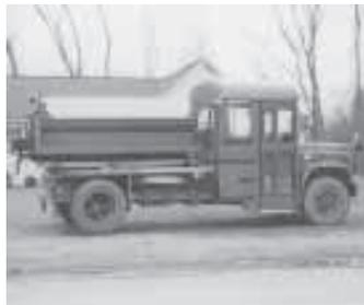
**To shorten the bus, Fry slid the wheels up and cut off part of the driveshaft. Then he cut 17 ft. off the frame on the back end.**
