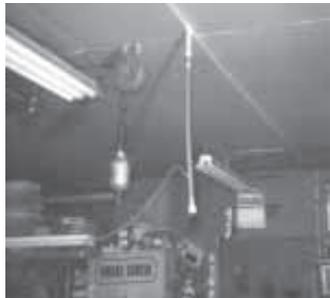
1/2-in. dia. PVC lines up one wall, along the ceiling, and down the opposite wall. An air compressor is hooked up to a 'T' coupler that's mounted on one wall. There's also a T coupler on the ceiling, with an air hose hanging down from it, and a coupler on the
