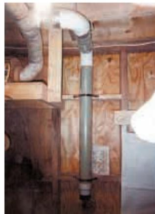
There are four connections to machines and an adapter for floor cleaning.
