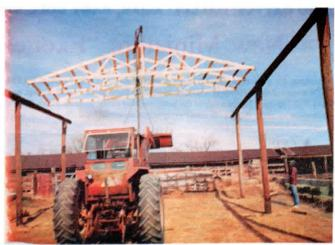
Miller makes Y-shaped brackets to mount crossbeam poles on top of upright poles. Then he uses boom to lift individual sections of three trusses each into place.
