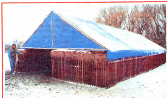
Alvis Beaver used flax big round straw bales to build this barn for 65 sows.
