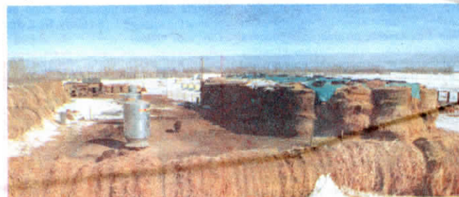
Alvis Beaver used flax big round straw bales to build this barn for 65 sows.
