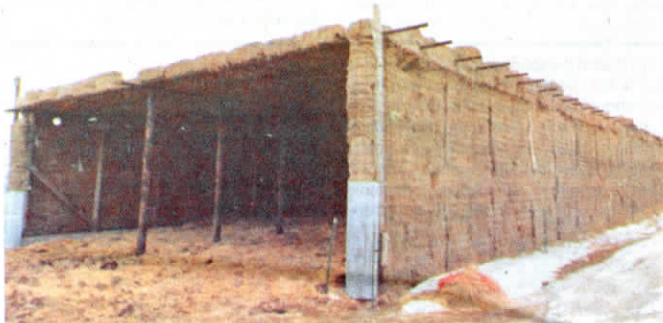
Greg Ankenbauer built two 40 by 120 by 14-ft. high cow calf straw barns.
