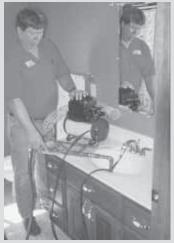
"Gunk remover" shoots compressed air into bottom of water heater via a hose connected to drain pipe. Air compressor hooks up to faucet.
