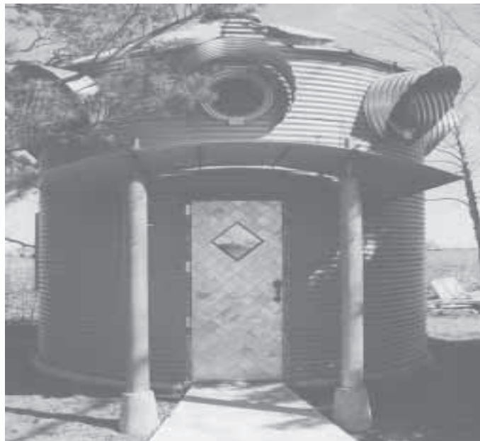
Architect Mark Clipsham turned this used 14-ft. dia. grain bin into a combination garden/storage shed and playhouse that’s complete with a second floor and a narrow spiral staircase. Note porthole-style windows all around.
