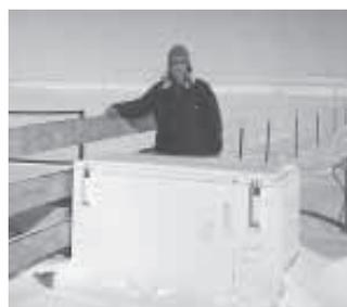
Gordon Kozroski uses an old chest-type freezer as a "pump house" to keep his water pump from freezing.
