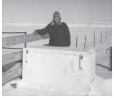
Gordon Kozroski uses an old chest-type freezer as a "pump house" to keep his water pump from freezing.
