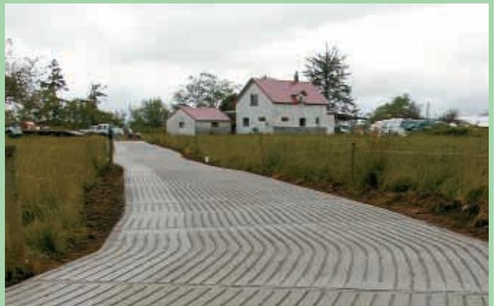
Oregon contractor Marty Richter lays concrete driveways and field walkways using a concrete version of the kind of "box" asphalt companies use.
