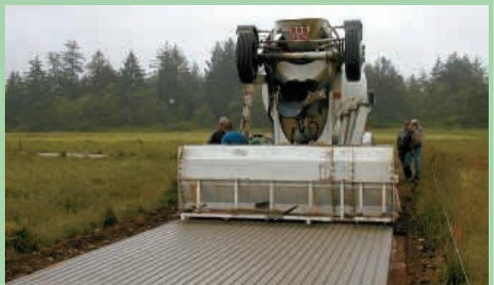
Concrete box lays strips from 5 to 15 ft. wide with 1/2-in. grooves every 4 in.
