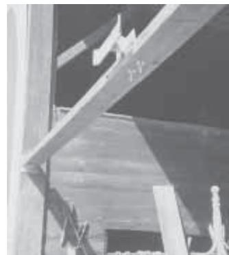
The two doors meet inside the bracket, which keeps the doors rigid so they can't blow either in or out.
