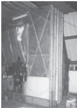
It consists of 4-ft. wide door panels, 10 ft. high. They slide along an old hay carrier track that Rick salvaged from a hay barn. Each door has a rolling hanger attached to its top center. Once stretched out flat, they form an insulated wall.
