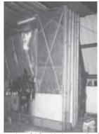
It consists of 4-ft. wide door panels, \$\overline{10}\$ ft. high. They slide along an old hay carrier track that Rick salvaged from a hay barn. Each door has a rolling hanger attached to its top center. Once stretched out flat, they form an insulated wall.
