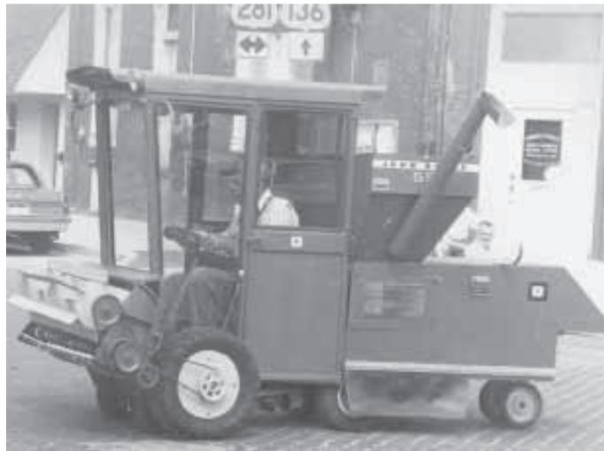
Pritts built this scale model Deere 55 combine on a Snapper riding mower. It has a cab, platform head, grain tank, working augers, and straw chopper.
