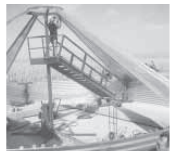
One master control raises all jacks at the same time, evenly and equally, so bin goes straight up.
