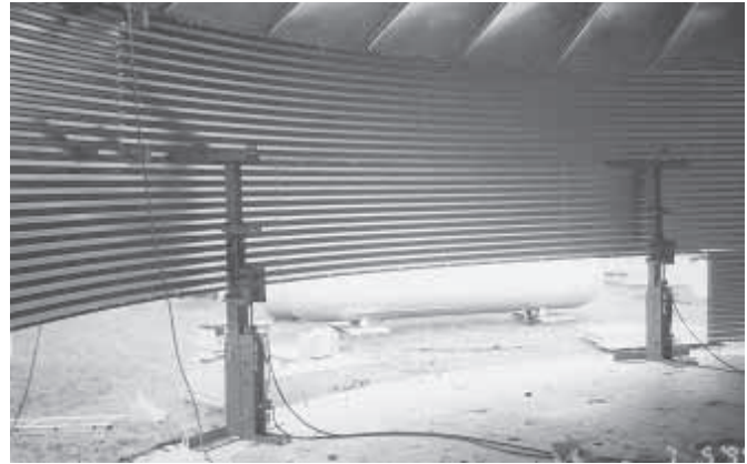
Jacks bolt to bin rings and can be adjusted for 32, 39 or 44-ring heights.
