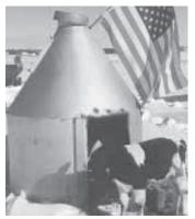
Hopper sets on ground upside down, with the top cut off and a door cut into one side.
