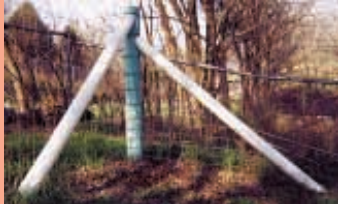
Concrete-filled PVC brace pipes are set at a 45-degree angle.
