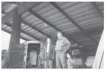
Lloyd Koos turned several 30-ft. long underground fuel tanks into beams and rafters to build this  $60\ by\ 60$ -ft. steel shed.
