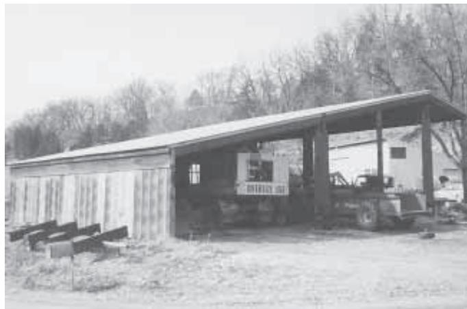
Koos cut strips of steel lengthwise and then welded them together in pairs to create relatively lightweight, oval-shaped steel "beams". Larger strips were cut for columns.
