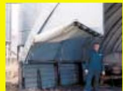
have been able to fit my 30-ft. self-propelled swather through the door, so when I put up the building I ordered it without the door framing members and built my own modified door frame. By hinging the door posts 7 ft. off the ground, I can flip up the canvas on both sides of the door so the header will fit inside the building.
