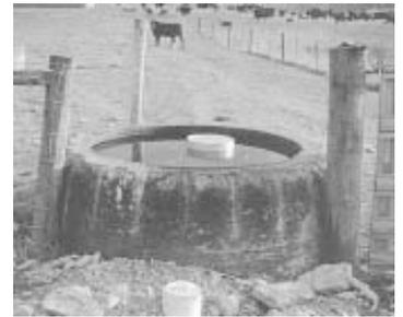
Center of tire is filled with concrete level with bottom bead on tire. After the concrete has hardened Bach installs the stand pipe, float system, and overflow.
