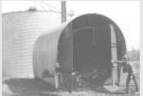
Taking a cue from high-efficiency wood stoves, Terry Greer of Arenzville, Ill., built his straw-burning furnace to be air tight, equipped with forced air draft and thermostatic controls. This enables him to precisely control air temperature entering his drying bin.
