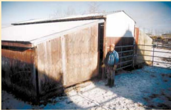
Greg Blahun built this 30 by 30-ft. barn in three sections, which are mounted on skids that make them easy to move around. Each section is 10 ft. wide and 30 ft. long.
