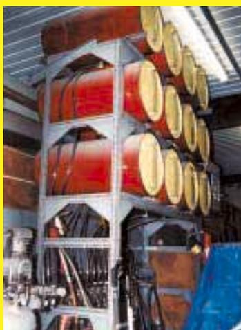
lets me see at a glance how much oil is left. Oil gravity-flows out of each tank through rubber hoses equipped with ball valves. Air pressure is used to pump oil up into the barrels. (John Imhoff, Rt. 2, Box 52, Roanoke, Ill. 61561 ph 888 817-5646 or 309 923-7345)
