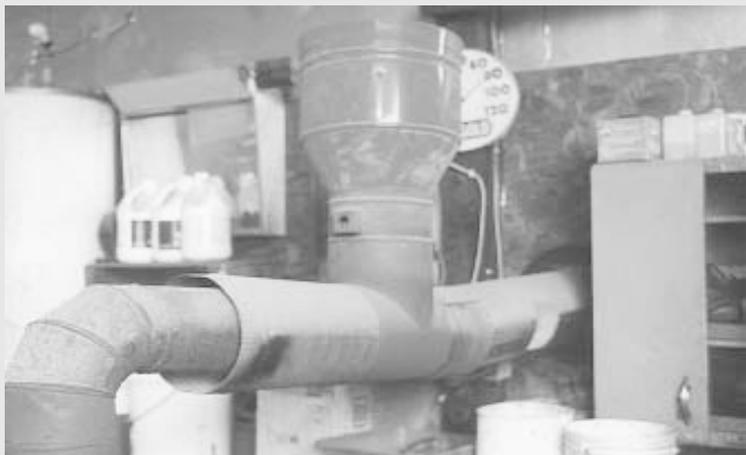
**Dunton slipped a large T-shaped section of pipe over the flue pipe on his stove. An aeration fan pulls heated air off the flue pipe and circulates it around his shop.**
