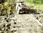
getting stuck so I made a heavy wood frame out of 2-in. planks. It lays flat on the mud so it can stand a lot of weight. I drove a steel post in at each corner and ran a light chain from the platform to each post to keep it from floating away when the water runs 3 to 4 ft. deep.
