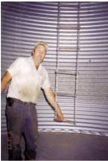
John Mason's chain-type safety ladder reaches down to within about 18 in. of bin floor.
