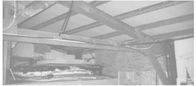
Poly tubing runs from Seubert's compressor up through the building's trusses to wall-mounted steel lines, which drop down to about 3 ft. above the shop floor.
