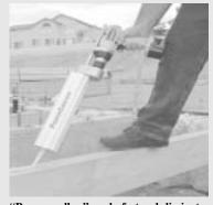
"Power caulker" works fast and eliminates the need for an air compressor.
