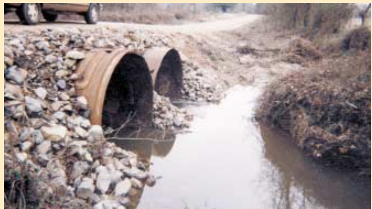
Tank car culverts are available in 7 to 10-ft. diameters and in lengths from 30 to 63 ft.
