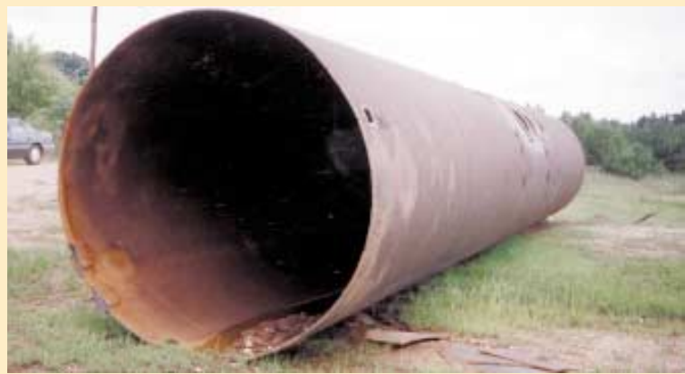
Old tank cars with the ends cut off make ideal culverts, says Terry Smith, who has been selling rail car culverts for several years.
