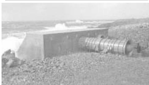
Back side of wave-powered electric generating station is fitted with a turbine. It's driven by air that's compressed by incoming waves.
