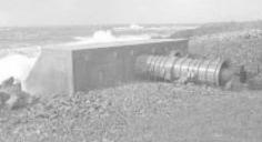
Back side of wave-powered electric generating station is fitted with a turbine. It's driven by air that's compressed by incoming waves.
