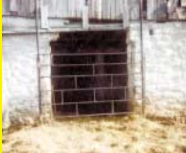
allow the gate to pivot. Adjustable chains run from the hinges up to swiveling rain caps on top of the pipe so the gate can be raised as needed to clear snow and manure. Anchor pins at the bottom of each end of the gate fit to the brackets. Small rods on the gate lock into the hinge brackets to prevent the gate from being lifted off by livestock. **(Harold Kirk, H-K Farms, Spring Bar, Manitoulin Island, Ontario Canada)**
