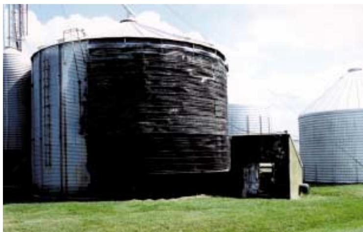
The Lortons built this passive solar collector panel around their Shivvers 10,000-bu. grain drying bin. Sheets of tin, painted black, run from under eave down to the ground.
