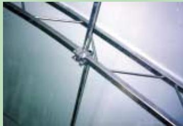
Trusses are made from square tubing, webbed together with solid steel bars.
