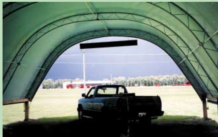
Stream Shelters welds its trusses together and then galvanizes the finished product. "That makes them far superior to other products which are galvanized first and then welded together. We treat the entire truss, including the welds," notes Darryl.
