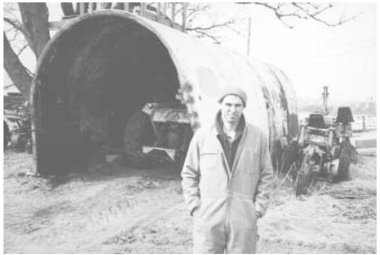
Charles Ballinger built this low-cost machine shed out of two salvaged gas tanks and a liquid fertilizer tank. The three 12-ft. dia. tanks are butted together end to end.
