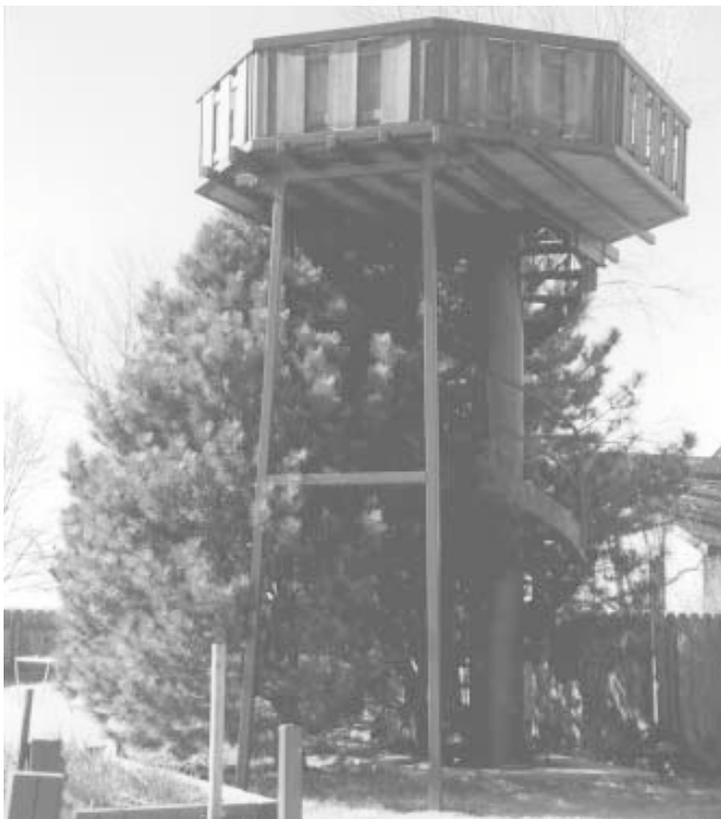
Deck perches 20 ft. above ground, with a 72-in. dia. spiral staircase leading up to it from below. Support is provided by a 24-in. dia. steel pipe and a pair of steel legs.
