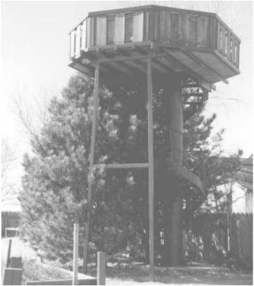
Deck perches 20 ft. above ground, with a 72-in. dia. spiral staircase leading up to it from below. Support is provided by a 24-in. dia. steel pipe and a pair of steel legs.
