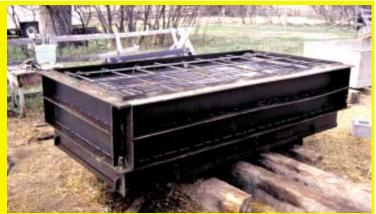
Photo shows steel forms set up with rebar and side panels around them, ready for concrete to be poured.
