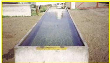
Boehmler made this 24-ft. long, 4-ft. wide trough by joining together three sections of precast concrete.
