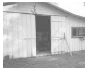
Bifold Dutch doors cover 16-ft. wide openings at either end of barn.
