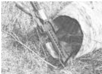
trucks cutting corners too short. To correct the problem, he modified a handyman jack with jaws to reshape the ends.
